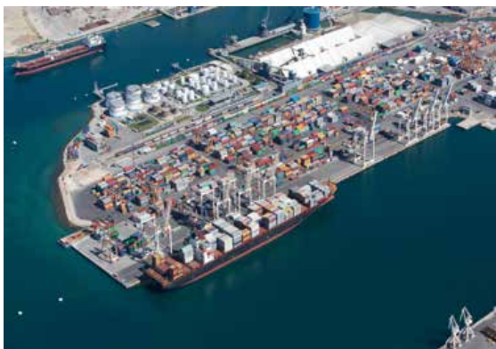
Upgrading the container terminal at Pier I
